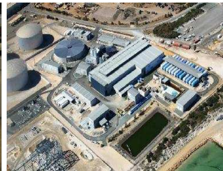
Perth Desalination Plant (Australia)
